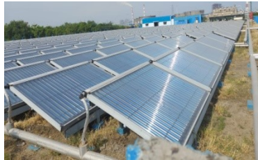
Fig 2: Solar Desalination Plant installed at NTECL
