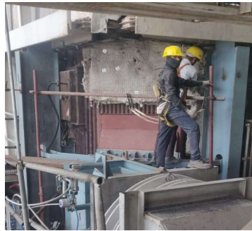
Fig 8: NOx reduction – combustion modification works in boiler
