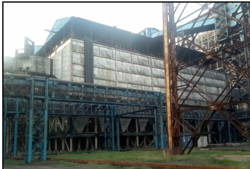
Fig 6 : Electro Static Precipitator at NTECL
