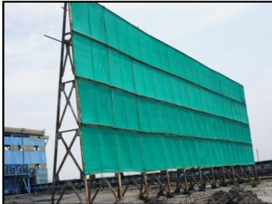
Fig 11: Wind barrier for coal stock yard at NTECL
