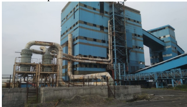
Fig 12: Dust extraction sytem at Coal crusher house
