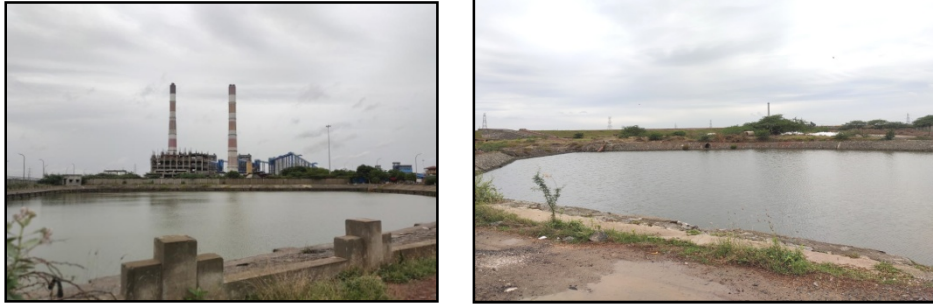
Fig 4: Rain water harvesting ponds at NTECL
