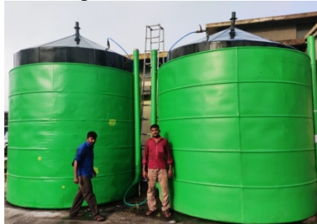
Fig 1: Installation of Biogas plant for canteen food waste at NTECL Plant
