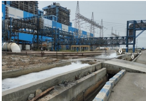
Fig 5: Main Drain separation construction completed in 2021-22
