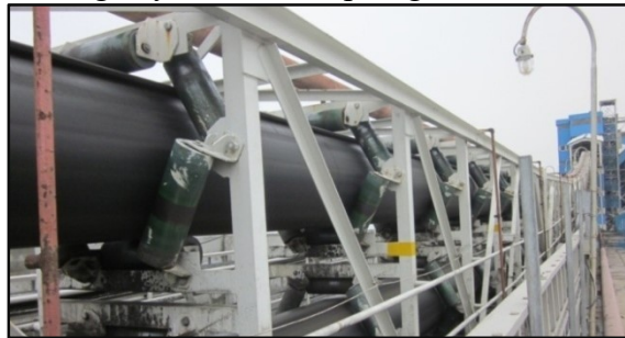
Fig 3: Pipe conveyor for Coal at NTECL
